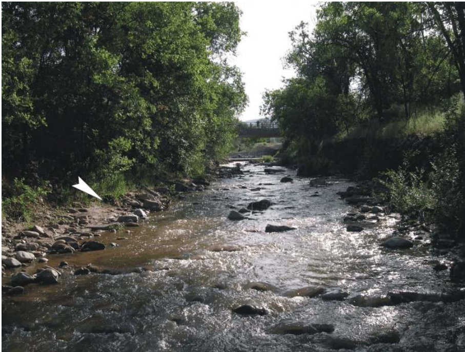
Figure 12. Stream type B4 below Camino Alire bridge. Arrow indicates field determination of bankfull stage. View is upstream, with the bridge in the background. Photo by J. Pittenger, 28 May 2007.
