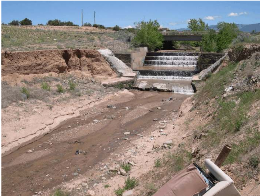
Figure 21. Grade control structure GCS-2 at the CR 62 crossing. View is upstream. Photo by J. Pittenger, 24 May 2007.
