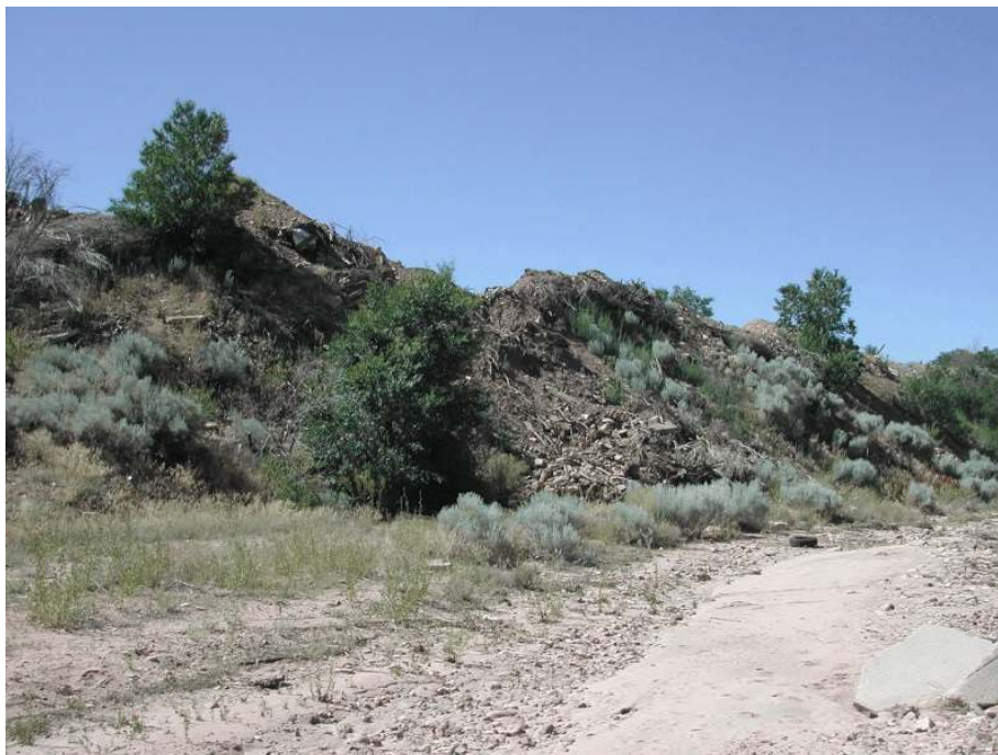
Figure 46. Waste piles spilling into the river channel. View is downstream in the reach below Camino Carlos Rael, 22 June 2007. Photo by J. Pittenger.
