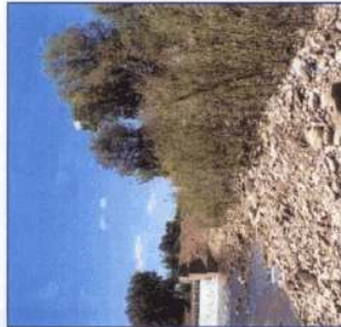
Before and after. Streambank stabilization is achieved by "deep planting" coyote willow whips; planting holes were augered in the rocky soil by using rotary hammers.
